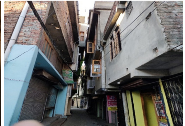
Construction without set-backs in main bazaar area of Chamba (05.12.2019)
