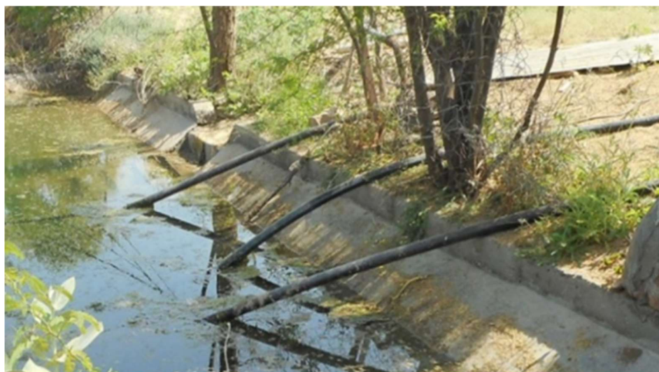
Unauthorised water lifting in NCP as water was taken directly from canals
