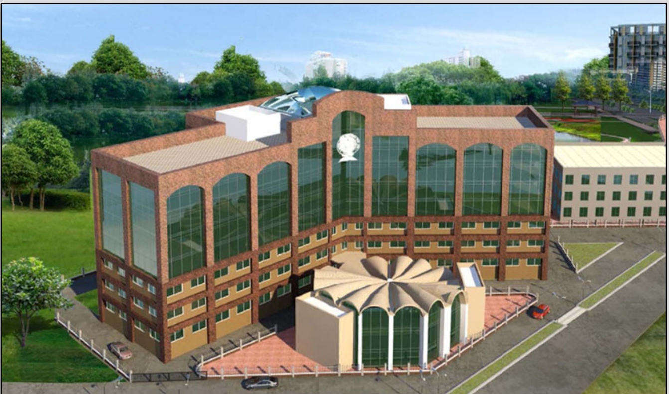
New Academic and Administrative Building of IIPS (under-construction)
