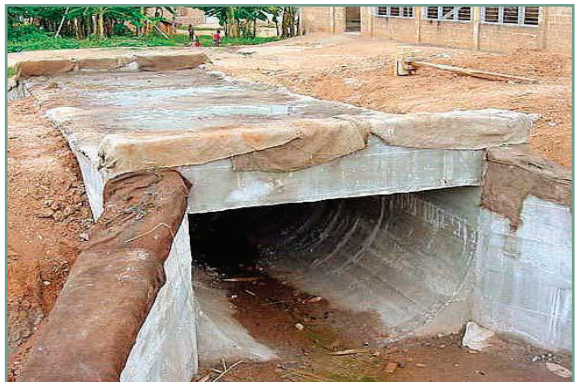
Figure 24: Curing of concrete with wet gunny sacking
