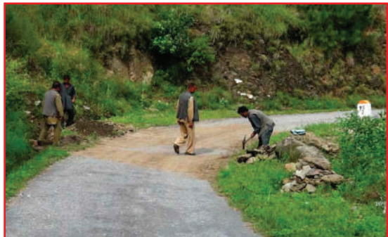
Figure 8: Workers performing routine maintenance
